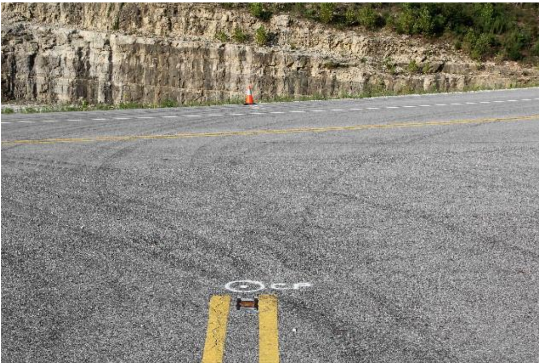
Figure 3: View of the southbound centerline at intersection with eastbound road
