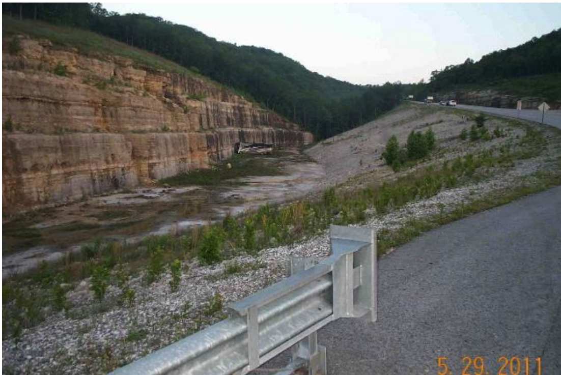
Figure 2: View from the east of the vehicles at POR
